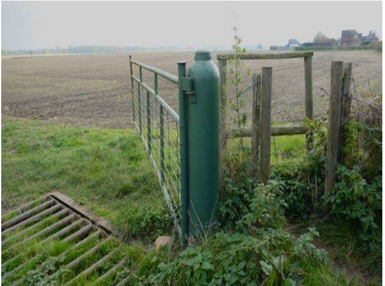
Figure 19: Gas cylinder gate post at Chilmington Green, retrieved from RAF Ashford 1945 (Photo: Ian Wolverson)
