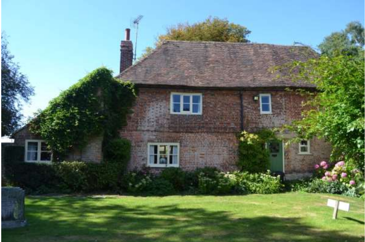
Figure 8: Farmhouse in the east of the borough - hipped roof with clay tiles; red brick and timber casement windows, typical of this area.
